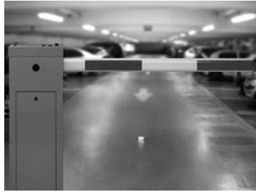
ATV12 drive controlling an access barrier
