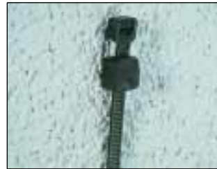
3. Place cable tie through mount.
