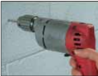
1. Drill hole using correct size bit.
