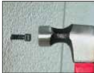
2. Hammer mount into hole.
