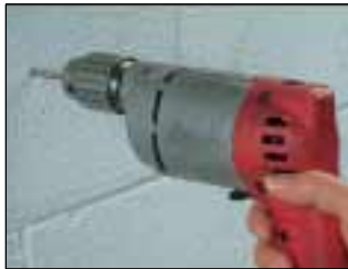
1. Drill hole using correct size bit.
