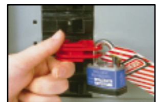
Verify that the lockout device secures the disconnect in a safe or off position.
