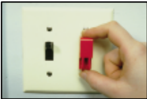
Lock out toggle switches without removing faceplates screws
