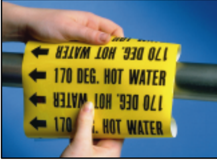
1. Spring open desired pipe marker.
