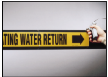
3. Secure strap snugly around the pipe, tension and cut the tie using Panduit recommended tool.
