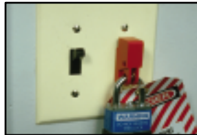
Lock out toggle switches without removing faceplates screws
