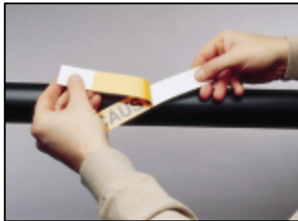
2. Separate the pipe marker from the liner.
