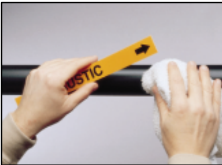
1. Clean the pipe with an appropriate cleaner and allow to dry.
