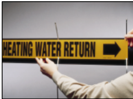
2. Place the marker against the pipe. Be sure the directional flow arrows are pointed in the proper direction.
