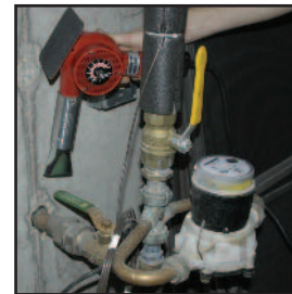
Thaw Frozen Pipes
