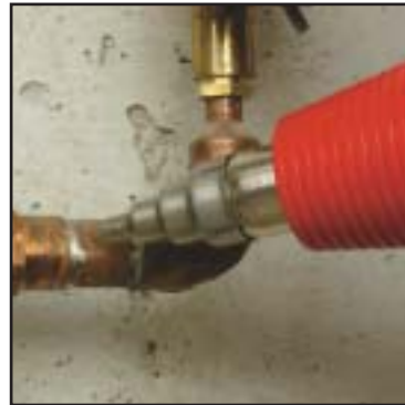
Solder Copper Pipe
