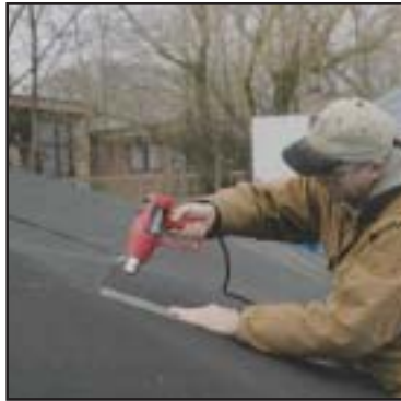
Weld Roofing Felt
