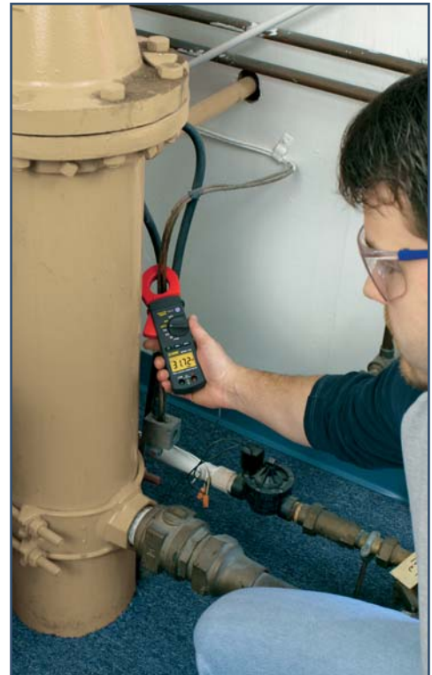
Measuring leakage current on a ground wire with the TRMS Leakage Current Meter Model 565
