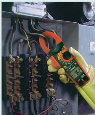
True RMS Clamp meter gives you accurate readings of non-sinusoidal waveforms
