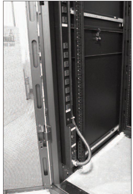
6B21N Power Commander Plus Power Distribution Unit shown mounted in an IT cabinet.
