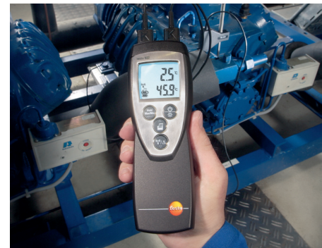
Simultaneous measurement of overheating and undercooling in refrigeration plants
