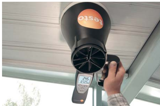
Using the testo 417 to monitor the air input at a ventilation outlet
