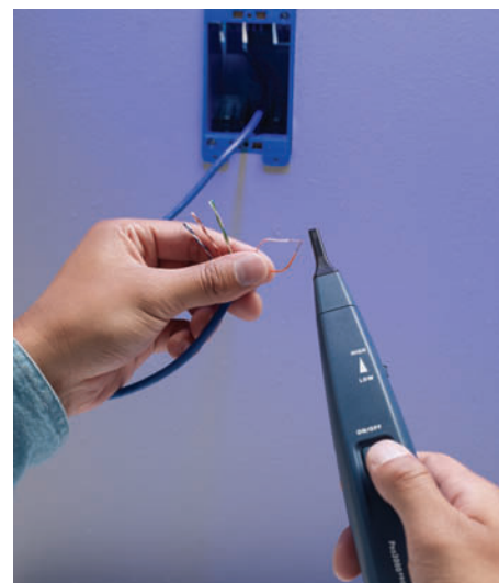
Hear the tone change when you short the correct pair on the far end
