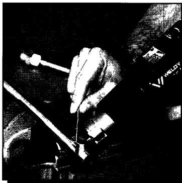
Soldering of copper pipes
