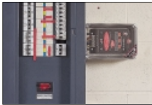
An ESP 415 M1 mounted, within a WBX 4 enclosure, directly alongside a mains panel and connected to its first outgoing way. Note how the protector is mounted on its side to help keep its connecting leads as short as possible.
