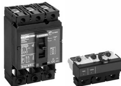
H-frame with Field Installable Trip Unit
