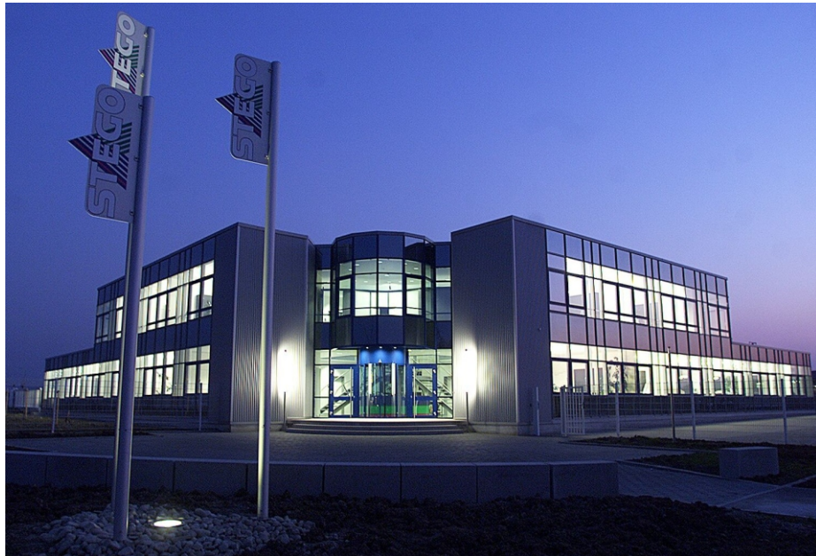
Photo: STEGO International Headquarters in Germany
