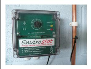
The Envirostat FP6i is an electronic thermostat designed to give energy efficient frost protection to pipe work where thermal insulation alone cannot protect pipes from freezing or being damaged by ice. With the cost of energy and the environment becoming a major factor that all businesses are now accountable for, United Automation has introduced the Envirostat range of
