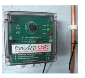
The Envirostat FP6E is an electronic thermostat designed to give energy efficient frost protection to pipe work where thermal insulation alone cannot protect pipes from freezing or being damaged by ice. With the cost of energy and the environment becoming a major factor that all businesses are now accountable for, United Automation has introduced the Envirostat range of products.
