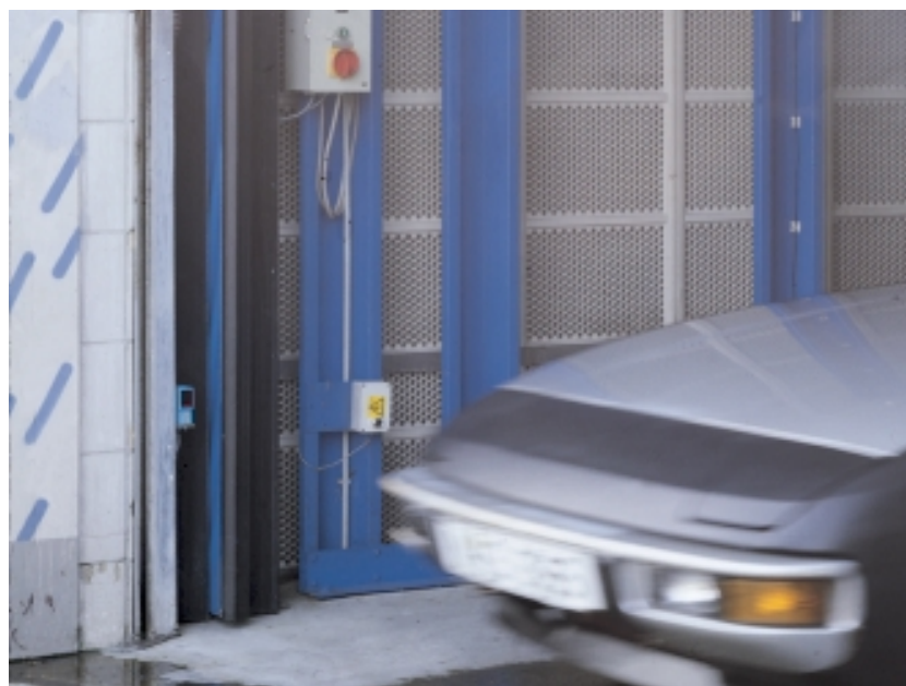
► Hot or cold, wet, dry or dusty – WL 36 photoelectric reflex switches are designed for use under hostile operating conditions indoors and outdoors – here they are being used on the roll-up gate of a carwash.
