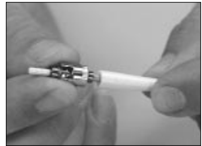
10.22 ST Connector—Install the boot on the connector.
