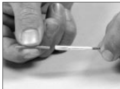
8.8 Remove the jacket from the end of the cable.
