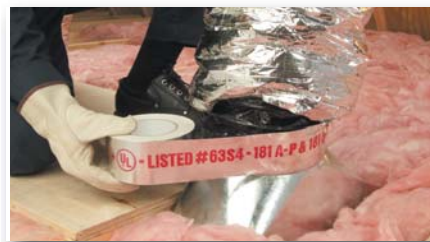
317 To seal fiberglass duct board and flexible duct systems, Scotch® Foil Tape 3326 meets the performance requirements for UL 181A-P and UL 181B-FX.
