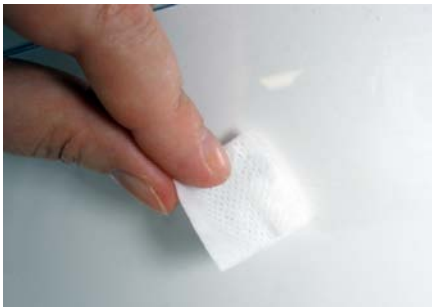
Figure 18. Adhesive Mount Antenna – Step 1. Pre-clean the surface
