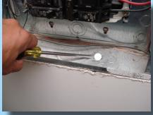
Using the screwdriver, remove panel knockout.
