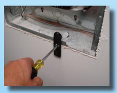
Push to loosen the knockout.
