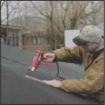
Weld Roofing Felt
